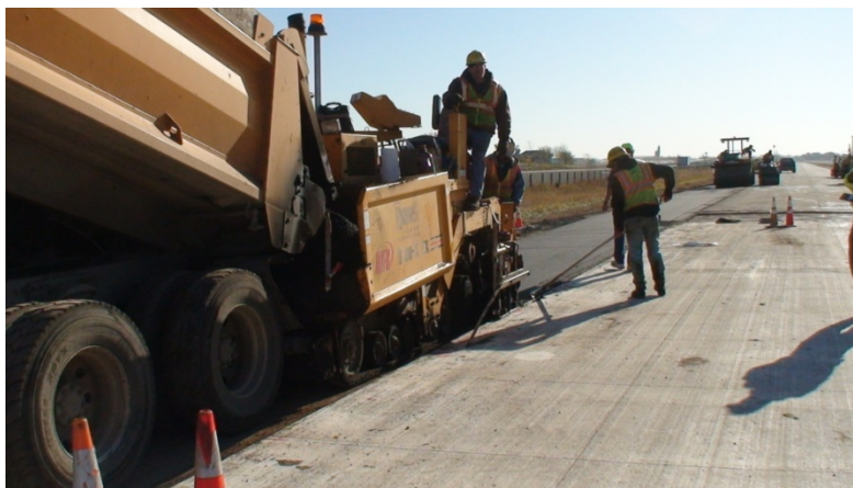
Figure 5.6. MnROAD MWSS Shoulder Construction
